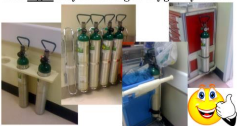
The right way to store gas/oxygen cylinders
